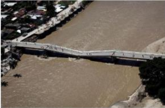
Figura 10 Colapso puente Coyuca I (SCT, 2014)
