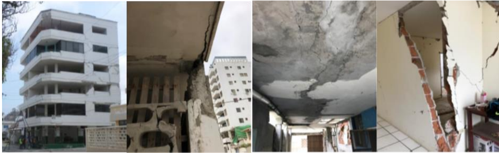
Figure 15. The Building Zedeño; (a) After The earthquake; (b) Damage in columns; (c) Crackings in panel of slab; (d) Collapse in masonry.
